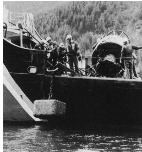
Figure 512. A sinker used to anchor a buoy.
