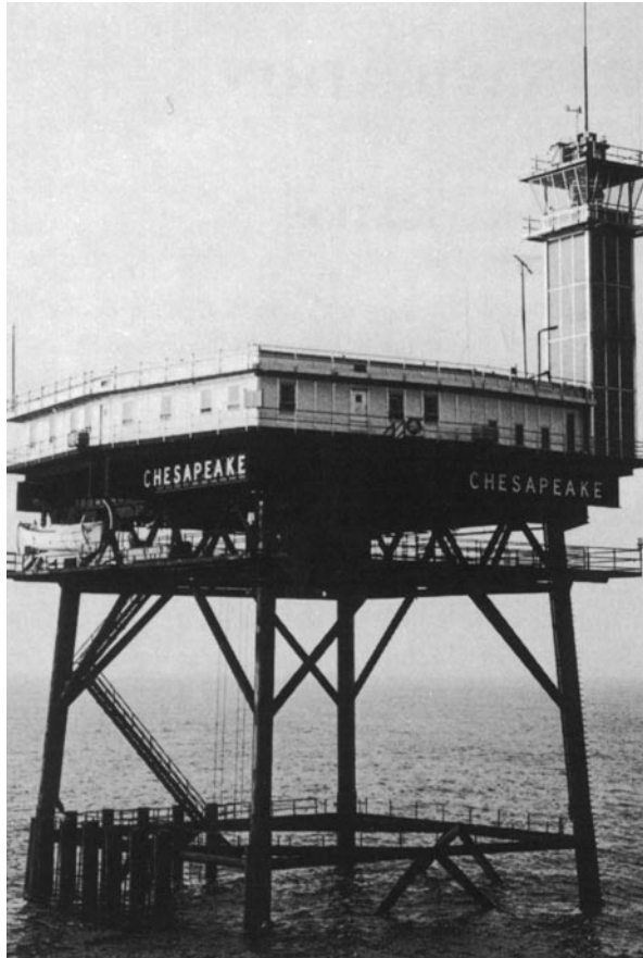
Figure 501a. Typical offshore light station.
