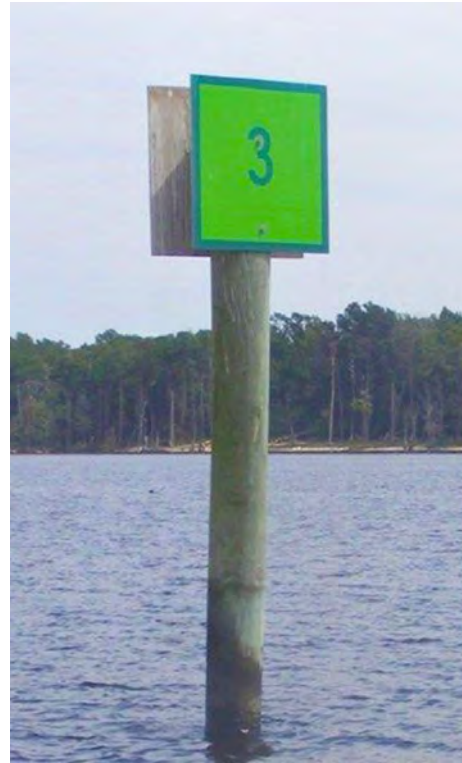
Figure 815. Unlighted beacon.
