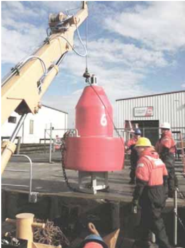
Figure 701b. Small lighted buoy.
