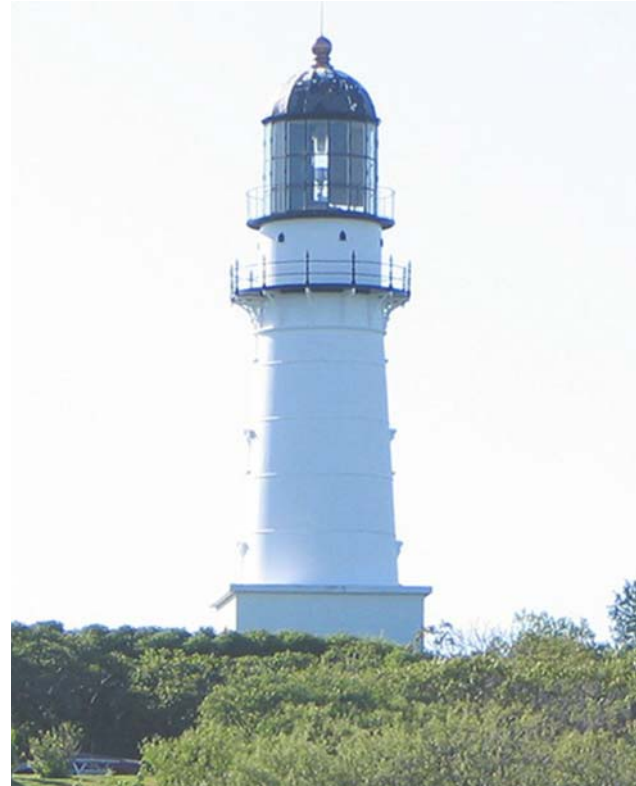
Figure 712. Typical Major Light.
