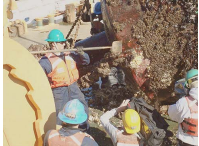
Figure 709. USCG removing marine growth from a buoy.
