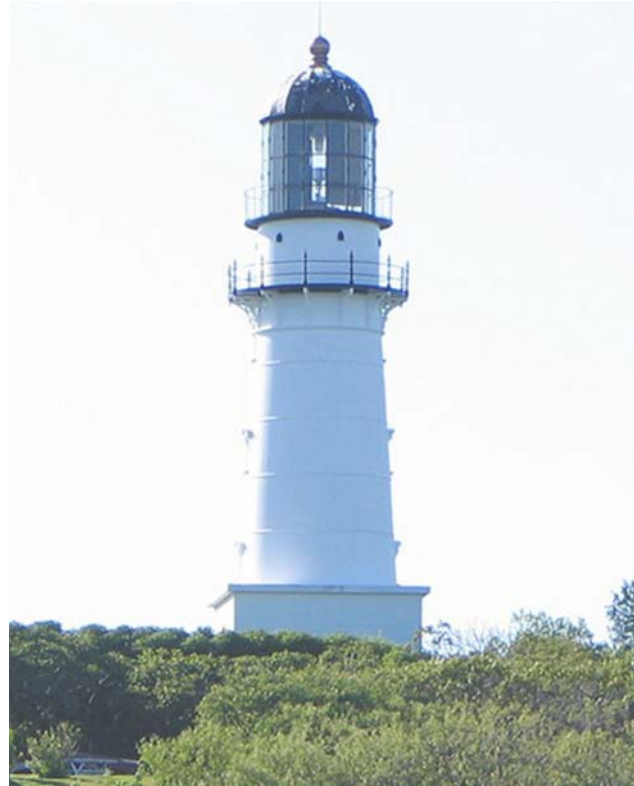
Figure 712. Typical Major Light.
