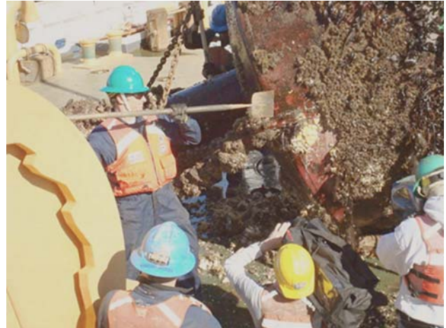
Figure 709. USCG removing marine growth from a buoy.
